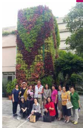
Under the cooperation of community residents, green vegetation is applied to the roof and façade of the community activity center. The indoor temperature of the center is effectively reduced by 5 degree Celsius.
